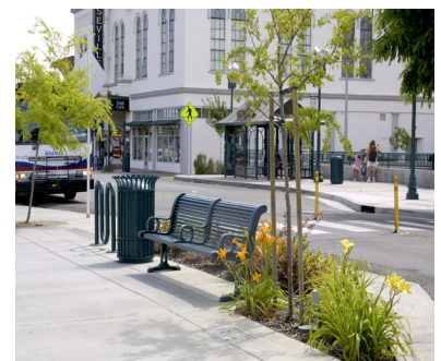
Lighting, signage, and street furniture on Riverside Avenue will be consistent with Vernon Street
