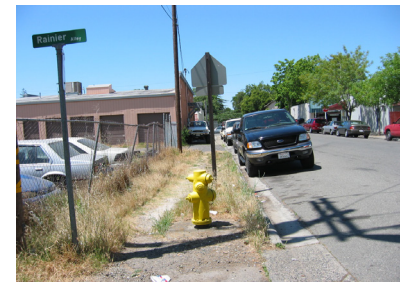
Sidewalk conditions vary throughout the Plan Area
