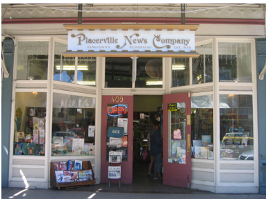
Use of large display windows at the street level
