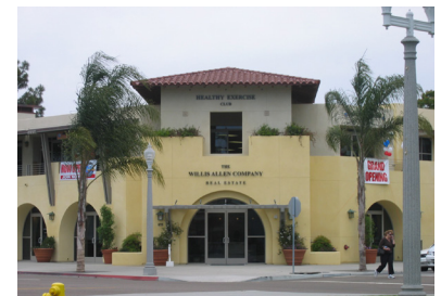
Example of appropriate building materials - stucco
