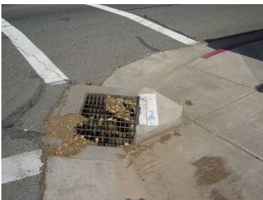
Existing storm drainage conditions on Riverside Avenue
