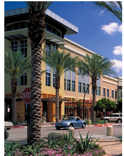
Examples of well-designed mixed use buildings
