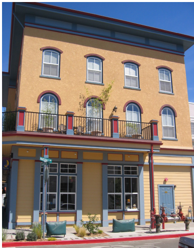
Example of a building with appropriate windows. The lower level has display windows while upper residential floors have smaller windows with approximately a 1:2 width:height ratio. All windows have clear glazing and mullions details
