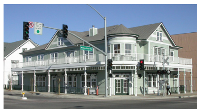
Building frontages feature display windows, entries and other human scale features
