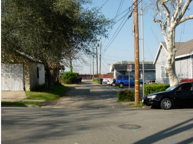
Existing overhead utility lines in the alleys within the Plan Area
